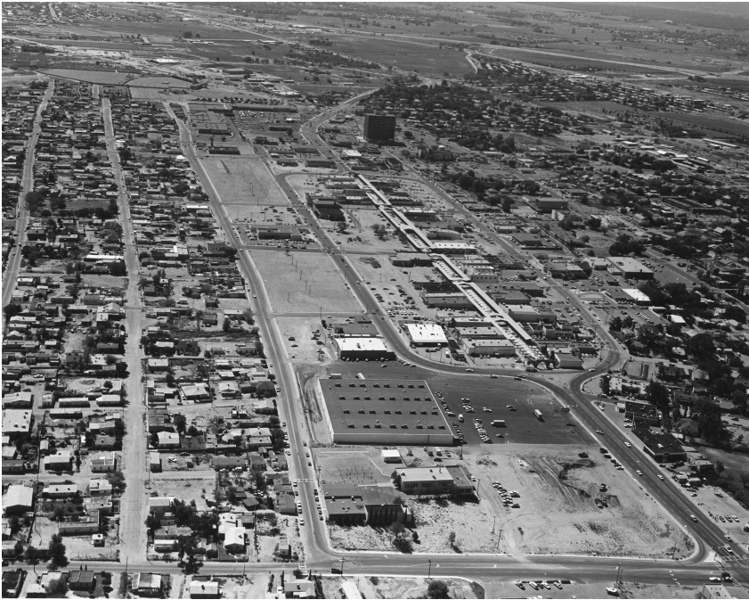
Fig. 1. Downtown Las Cruces in 1973 Looking South towards El Paso. This photograph captures the urban renewal peak. Main Street is turning into a pedestrian thoroughfare with a canopy, and the city adds a race track for automobile passage. On the left, or east, of Main Street is the Mesquite Neighborhood, home at the time to a predominately Hispanic population and the homes cluster together with little foliage. To the right, or west, of Main Street is the Alameda Neighborhood where affluent white Las Crucesians reside in homes on large lots. The original Bellamah Addition is just out of sight in the top left corner. Photo courtesy of the Las Cruces Urban Renewal Agency Records, 1966–1974, MS. 0478, New Mexico State University Library, Archives and Special Collection.
